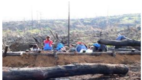
Fig. 2: Contour line dike implemented by Tencin University volunteers
