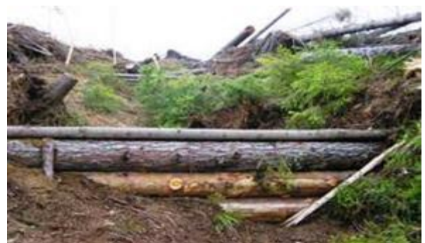
Fig. 4: Dike with timber wall implemented by Slovak Scouting
