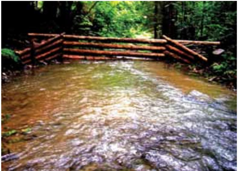
**Jednoduchá zrubová hrázka vzdúva hladinu vody v koryte a utlmuje jej silu na erodovanie dna koryta. | A simple log check dam raises the water level and dampens the energy of flow, which stops erosion in the river bed.**
