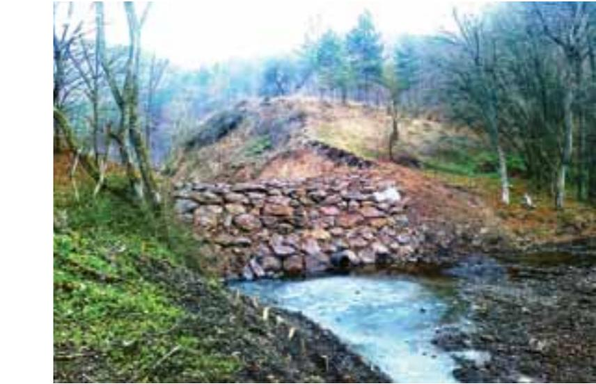
**Čiastočne obnovený 250-ročný tajch v Rudne nad Hronom s konštrukciou klínovaných balvanov, od roku 1929 poškodený.** | A partly restored 250-year-old pond in Rudne nad Hronom with construction of spiked boulders, that has been damaged since 1929.
