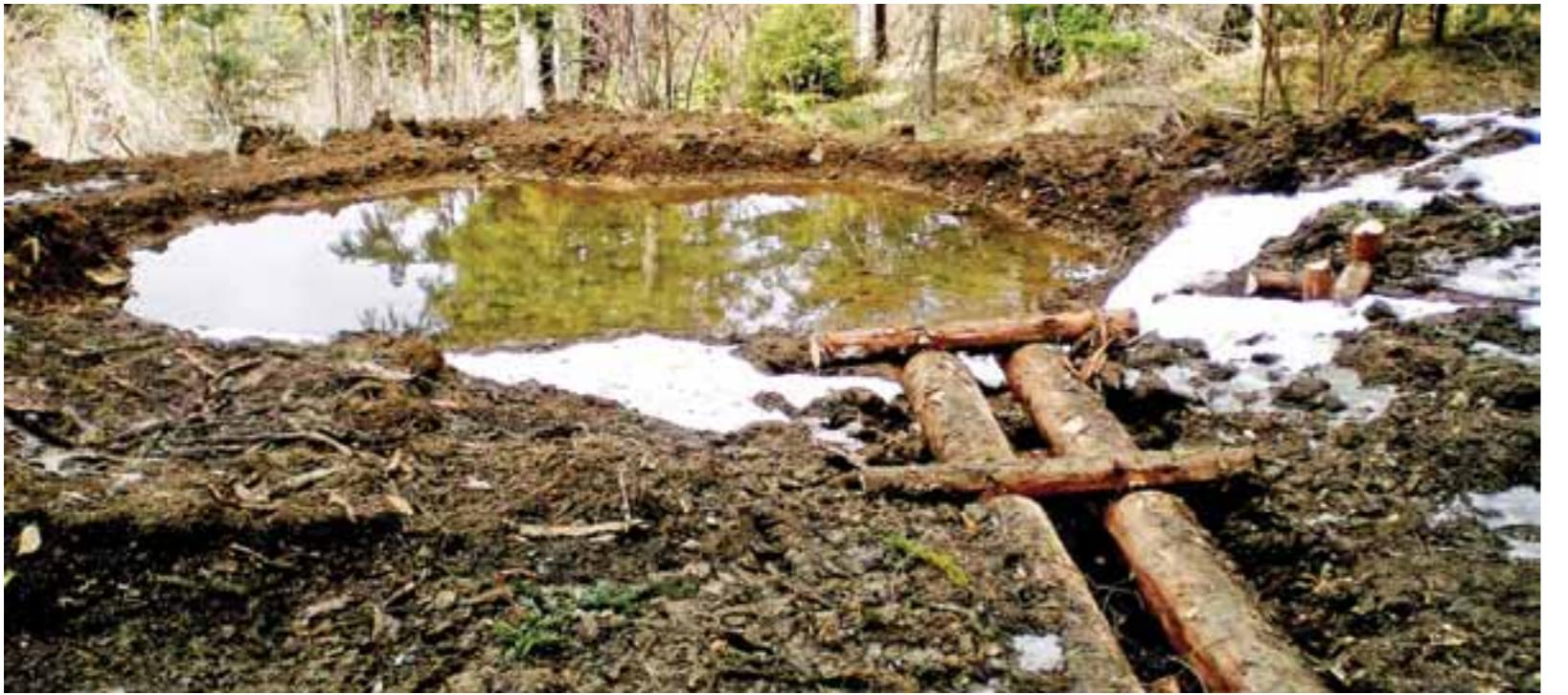
Takto funguje odrážka so zasakovacou jamou. | The performance of a surface cross drain with an infiltration pit.
