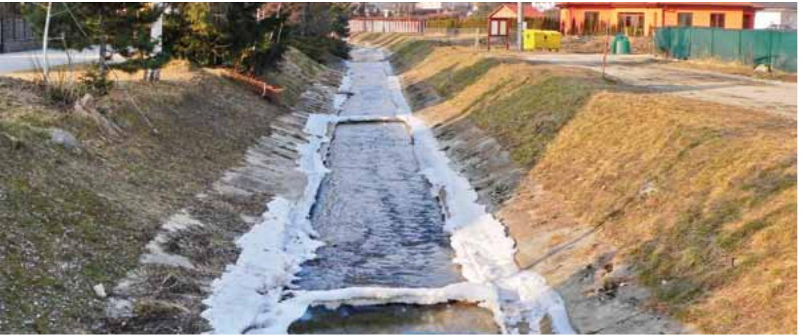
Zregulovaný potok v Dražkovicach je tiež vybudovaný na princípe posúvania povodňovej vlny „susedom na hlavu“. | Regulated and channeled stream in Drážkovice is build on principle of sending flood wave down on neighbours as quickly as possible.
