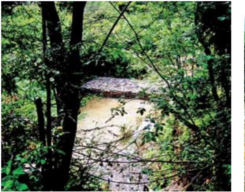
**Drôtokamenná hrádza vzdúva hladinu a priesakom čistí vodu.** | A gabion check dam made raises the water level and the water is cleared by its infiltration through stones.
