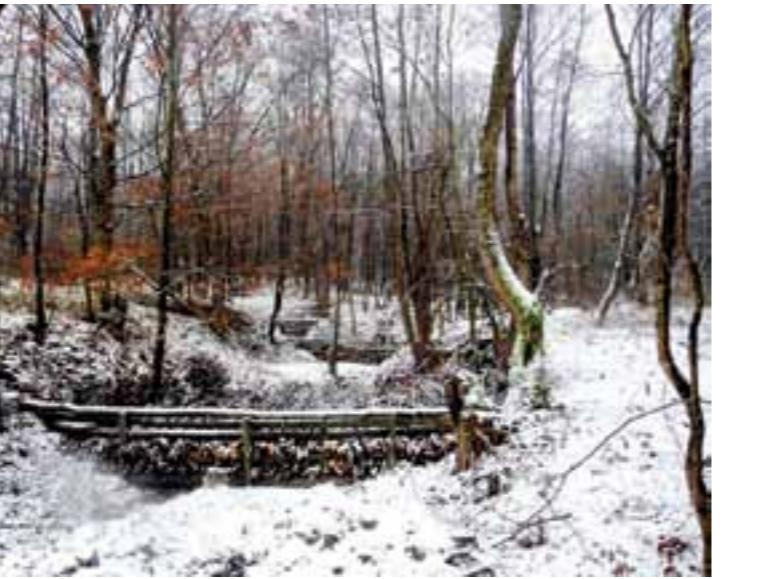
**Kaskáda drevených hrádzí sa postupne zanesie a zarastie.** | The cascade of wooden check dams will get gradually silted up and overgrown with vegetation.
