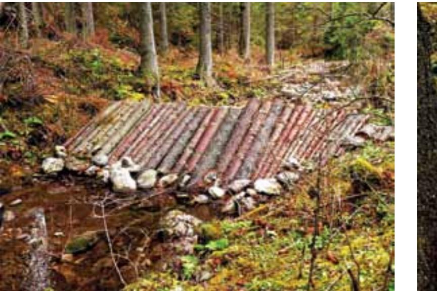
Kolové hrádze v Ždiari budú pomerne rýchlo zanesené sedimentmi. | The stake weirs in Ždiar will be relatively quickly silted up with sediments.
